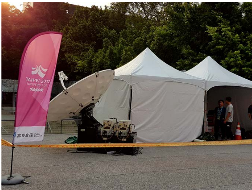
Globecast's new UHD-capable SNG equipment for 4K live transmission via AsiaSat 5
